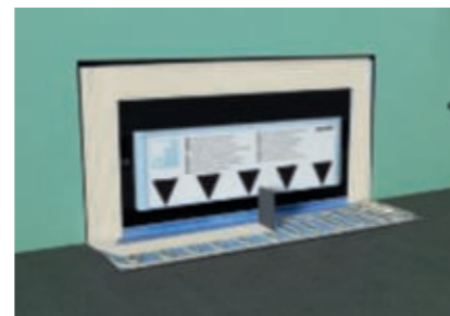
Cover panelling frame completely with glue
