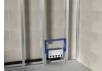
Connect discharge pipe
