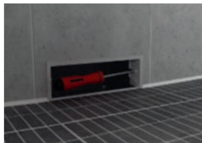
Install sight frame
