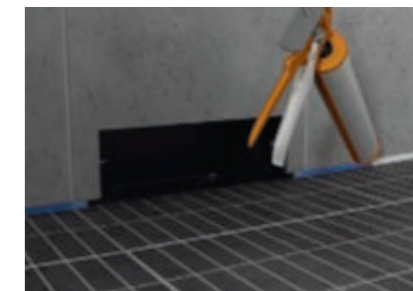
Lay wall tiles, then remove protection hood, apply silicone caulk
