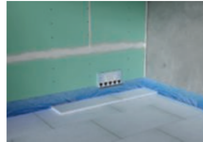
Lay thermal and impact sound insulation
