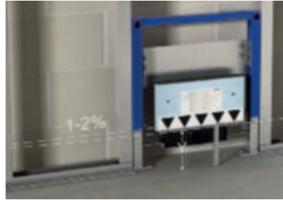
Adjust flange to screed height, observe 1-2% slope
